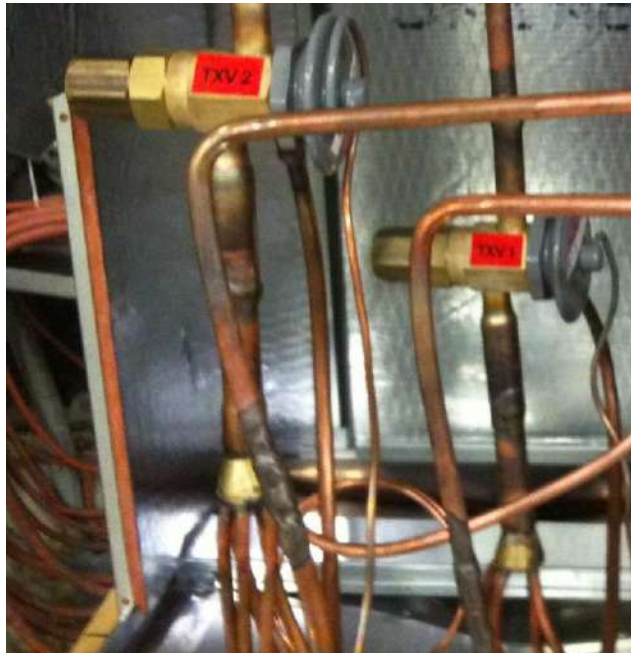
Thermal Expansion Valves
