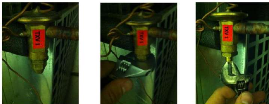
Figure 10 – TXV Adjustment
