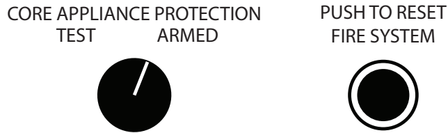
Figure 54 - Electrical Control Panel "Armed" Mode
